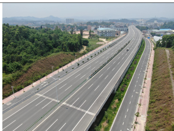
K51+800 两侧边坡采用喷播植草防护
